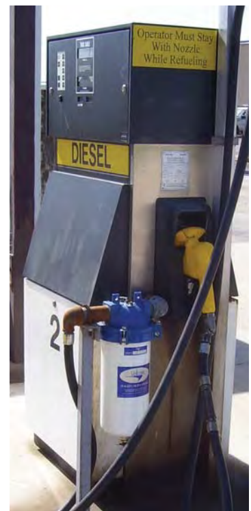
VF-61 connected to a diesel fuel dispenser
