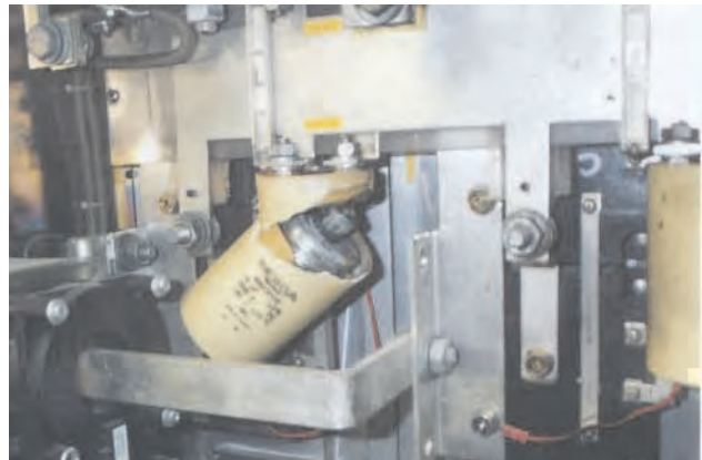
Photo 6, Capacitor Failure
